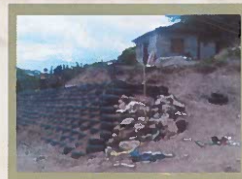
Tyre Soil Retaining Wall constructed in Metbrook Heights 2014
