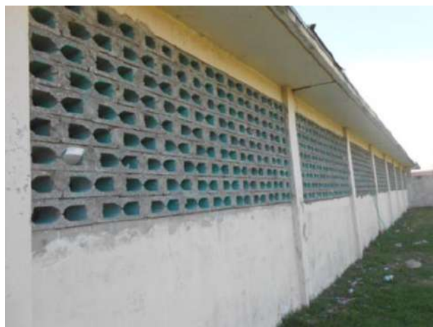
Fig: 1 Breather blocks in eastern wall that through which rain enters the shelter block before retrofitting
