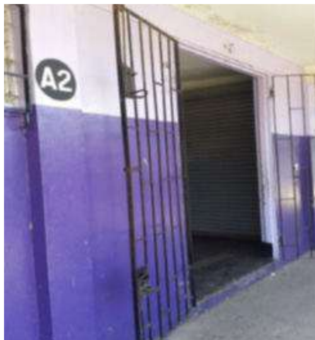
Fig: 2 Missing double-door on western wall of shelter block before retrofitting.
